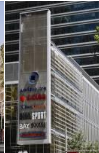
Sydney World Square Retail Complex and Public Car Park
